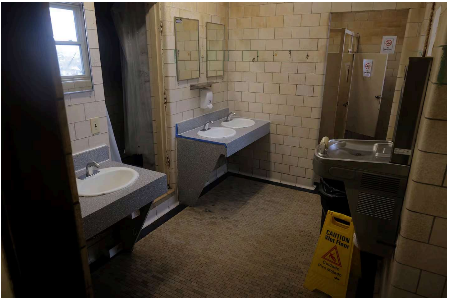
Residents in the Somerville YMCA's affordable housing units share communal bathrooms. LANE TURNER/GLOBE STAFF
